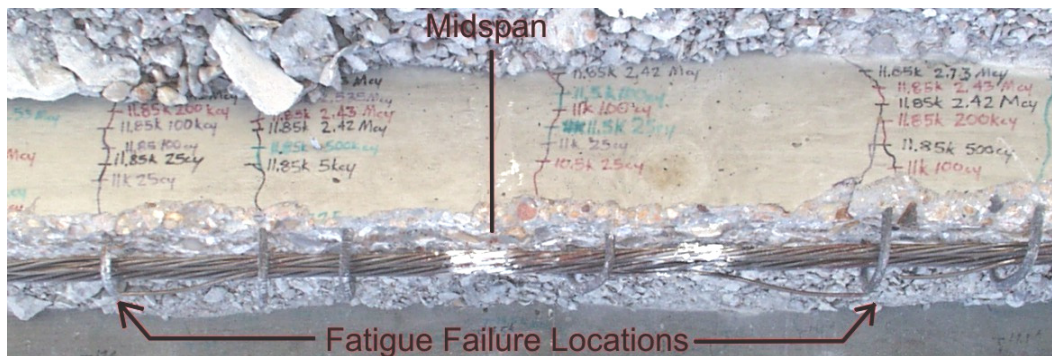
Figure 4-49 Photograph of Beam 3 After Removal of Concrete to Expose Strand
